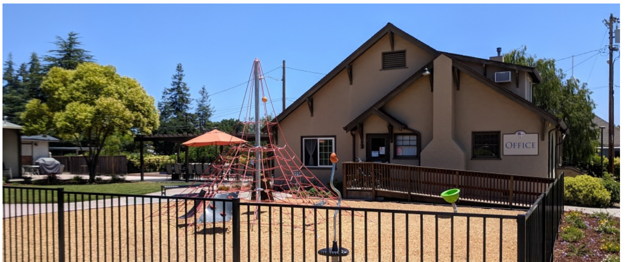
The parish office and new playground.
